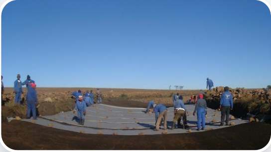
Crack sealing at Hlobane
